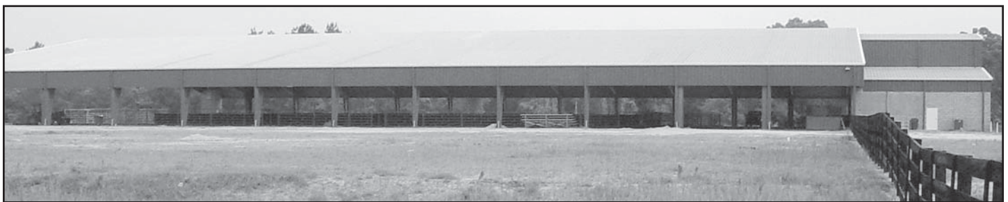
Side view of Wiregrass Arena building.
